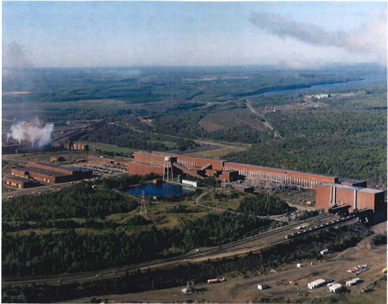
Figure 15. Erie Mining Company concentrator (right background) and coarse and fine crushers (right foreground); general shops and pelletizer at left, looking south, ca. 1999 (Polymet Mining).
